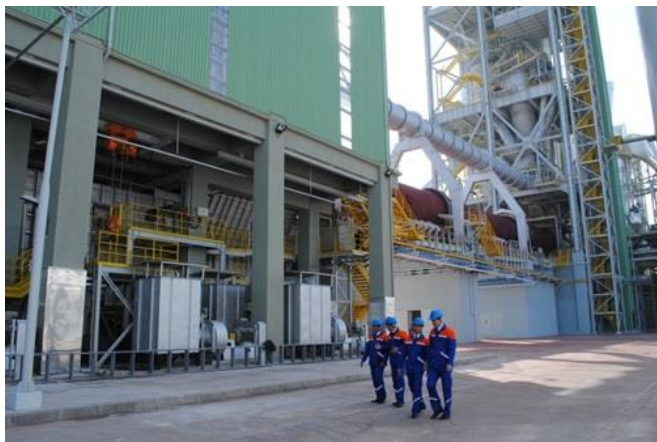
Picture 1 – The Construction and Industrial Complex
