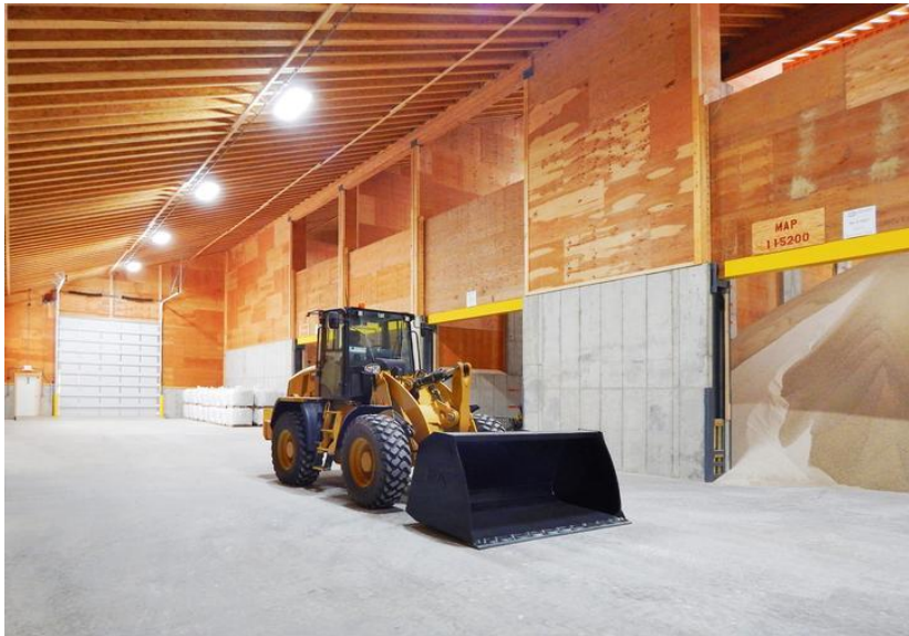
Figure 1 – Wooden glued arches of an unheated warehouse with a span of 30 meters.
